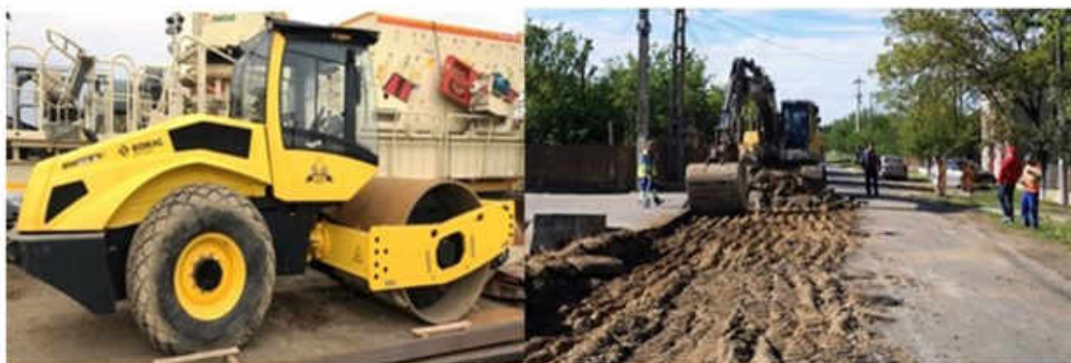
Figure 5. Road construction phase images – working with drum roller and excavator
