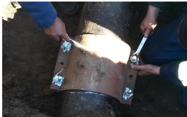
Image 1 - Generalized pitting located in the upper part of the pipe - totally destroyed external insulation (temporary repair)
